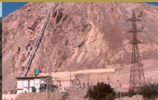
HIGH TENSION POWER LINES
