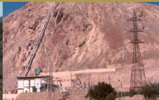
HIGH TENSION POWER LINES
